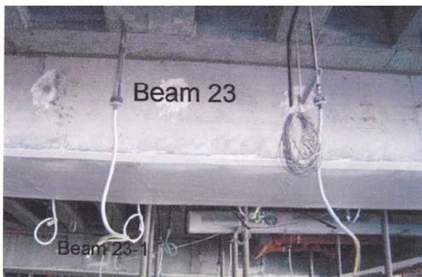
Fig 6: Carbon Fibre Plate at Beam
